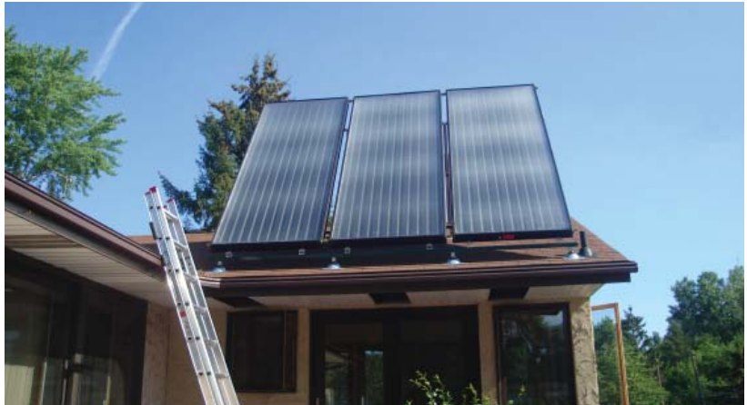
The "smoky" look of solar thermal panels and their thick black frames distinguish them from PV systems, but they can be similarly integrated into building architecture.
